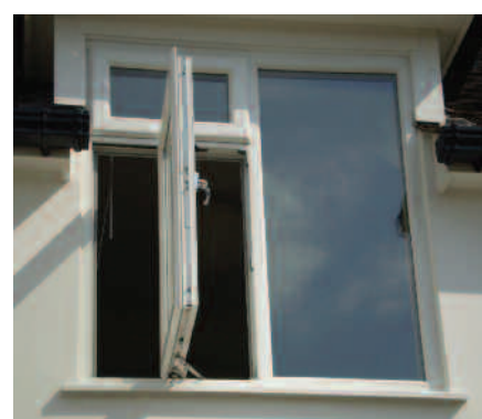
Easy Clean Hinges so that you can reach both sides of the glass to clean
